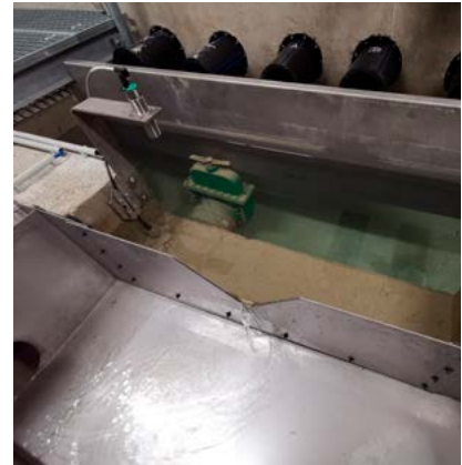
Seepage system of a dam with redundant flow measurement via ultrasonic and pressure level sensors.
